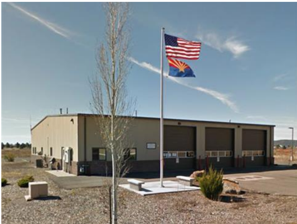
Figure 3: Street View of Existing Station
