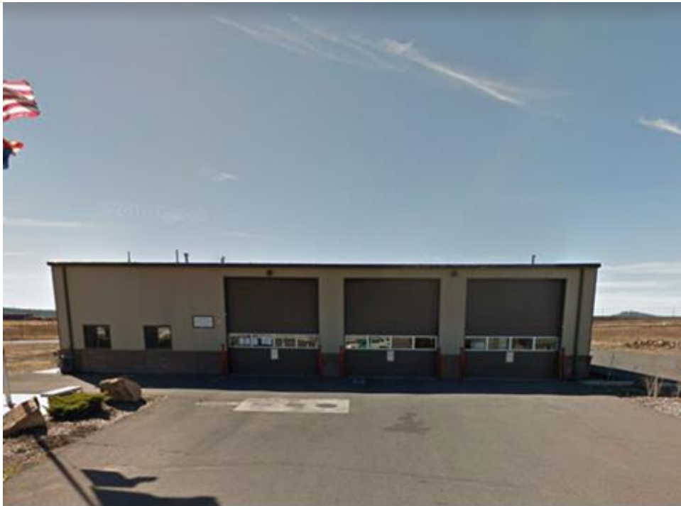
Figure 2: North Face of the Existing Station
